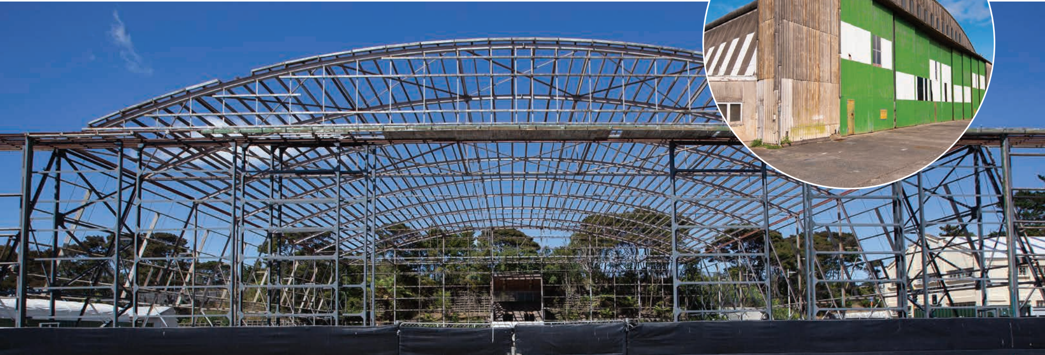
THE SUNDERLAND HANGAR, STRIPPED OF ITS ASBESTOS CLADDING
