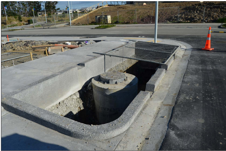
Correct Rain garden Edge Note - kerb higher than footpath
