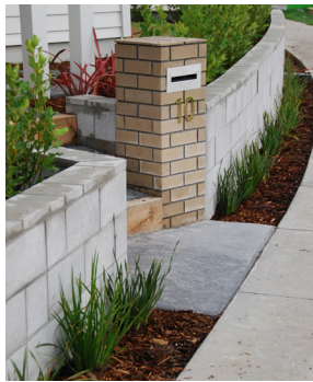
Concrete block retaining wall to front boundary with planting to screen.
