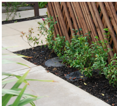
Service covers located in 600mm strip in front of fence, planting to screen.
