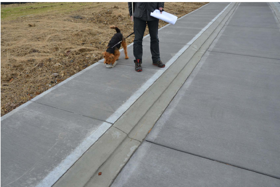
Correct Trowel Edge Detail - For edges parallel with carriageway
